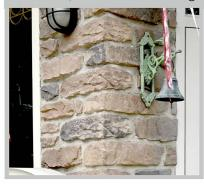
• Install the stones in a zigzag pattern to avoid creating any vertical straight lines.
