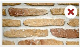
Ensure that the grout does not touch the stone's surface. If it does, wipe it off immediately with a damp cloth or sponge.
